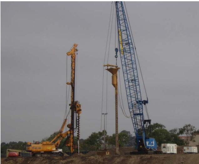
Fig 6. Equipment used for vibro stone column installation.
