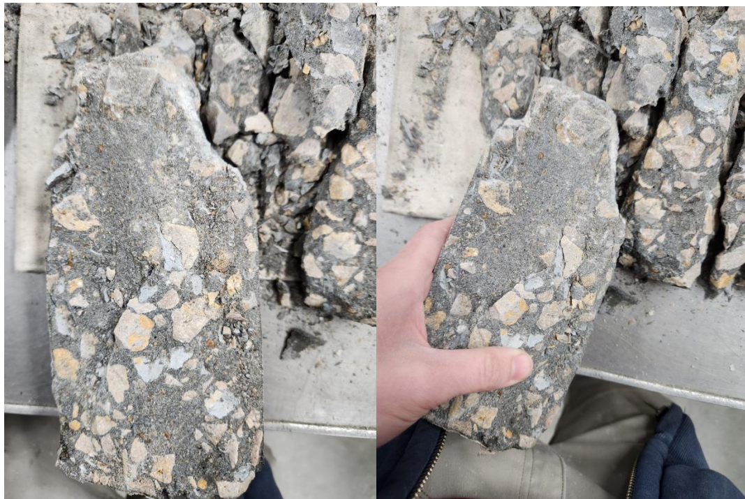
Figure 5.16 Cylinder Completely Broken
