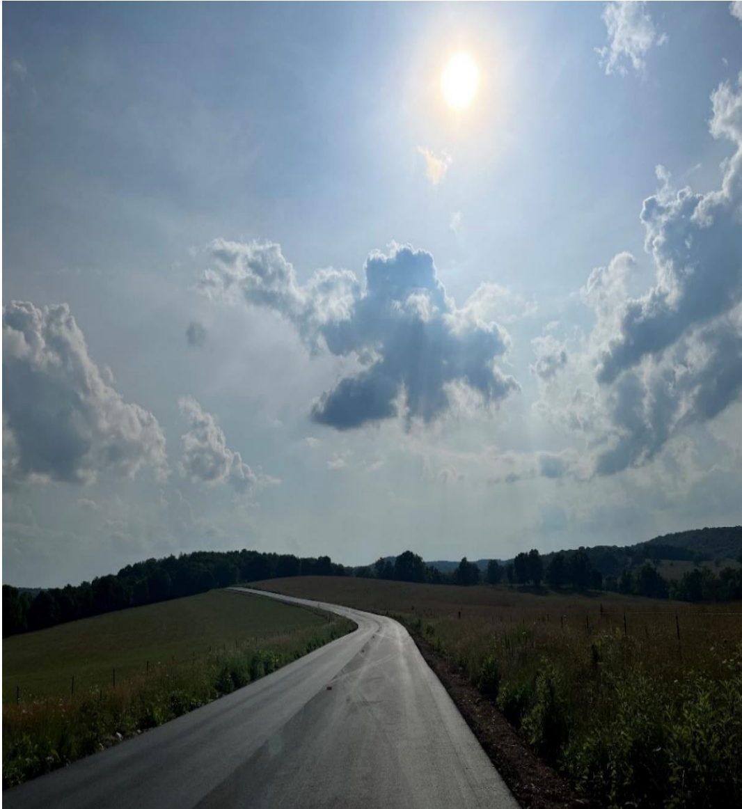
Figure 3.2 Snapshot of Route N (During Field Survey)
