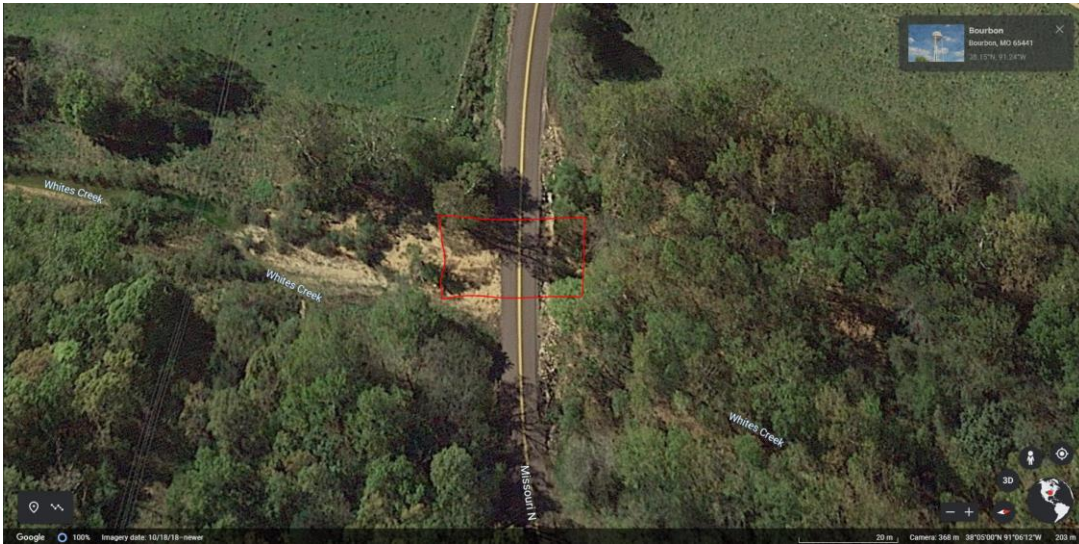
Figure 3.10 Whites Creek Crossing Route N (Area of Periodic Flooding).
