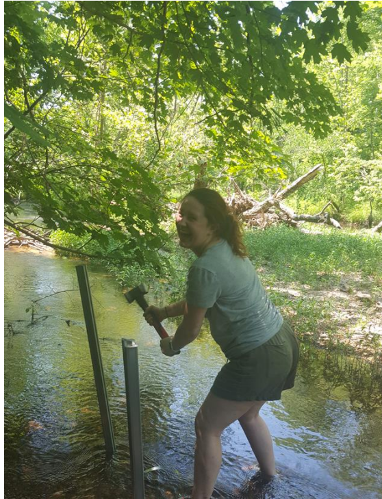
Figure 3.9 Installation of SuperStruts Into a Streambed by the Author, T.N. Mortensen.
