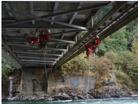
Figure 1.2. Rope Access Bridge Inspection [7]
