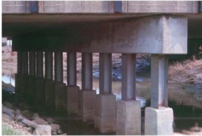
Figure 2.2: Concrete encasement repairing method (ODOT 2088).
