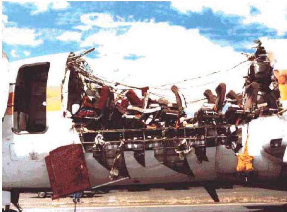
Figure 1-1 B737-200 N73711 Aloha Airlines Fuselage Damage Detail [2].
