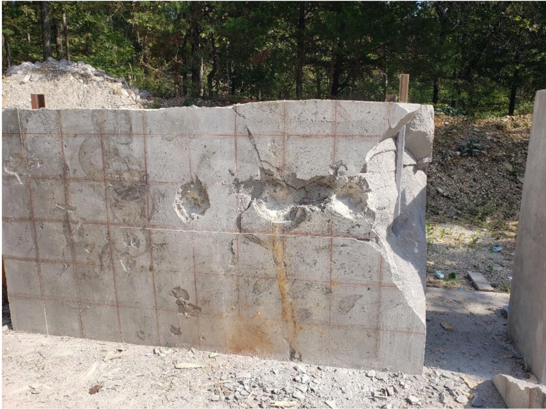
Figure 5.7 Unreinforced 50 psi Seal Damage
