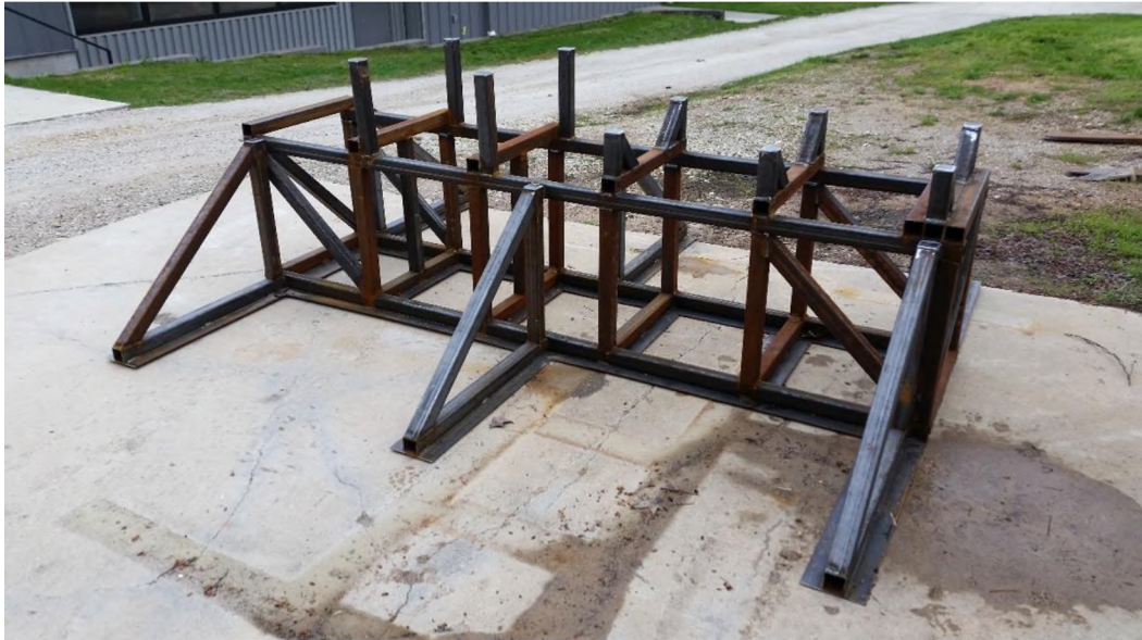
Figure 4.2 Frame During Construction
