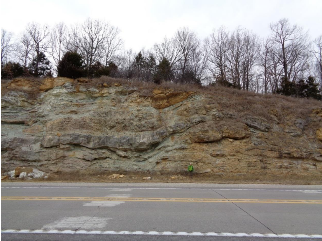
Figure 3.2. The “Cave Hill” road-cut on U.S. Highway 50 Missouri. Location of CZ-1 a well indurated sandstone in the older Cotter Dolomite and CZ-2 a more friable sandstone in the overlying Everton Formation is shown.
