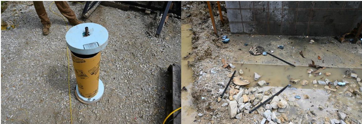
Figure A.63. Roof bolts
