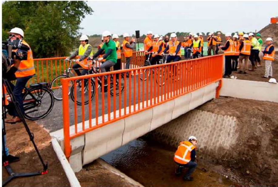
Figure 2.7. Implementation Example of 3D Printing: Pedestrian Bridge [6]
