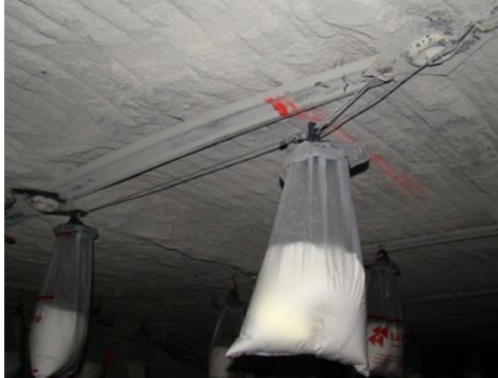
Figure 4.4: Cable and Hook Support Method
