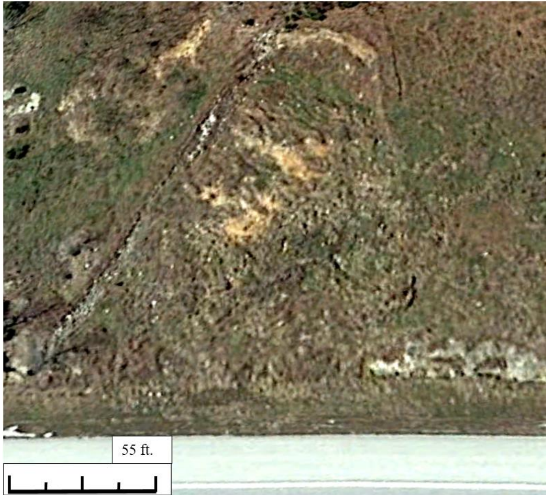
Figure 2.2. Google Earth Plan View of Stone County Landslide
