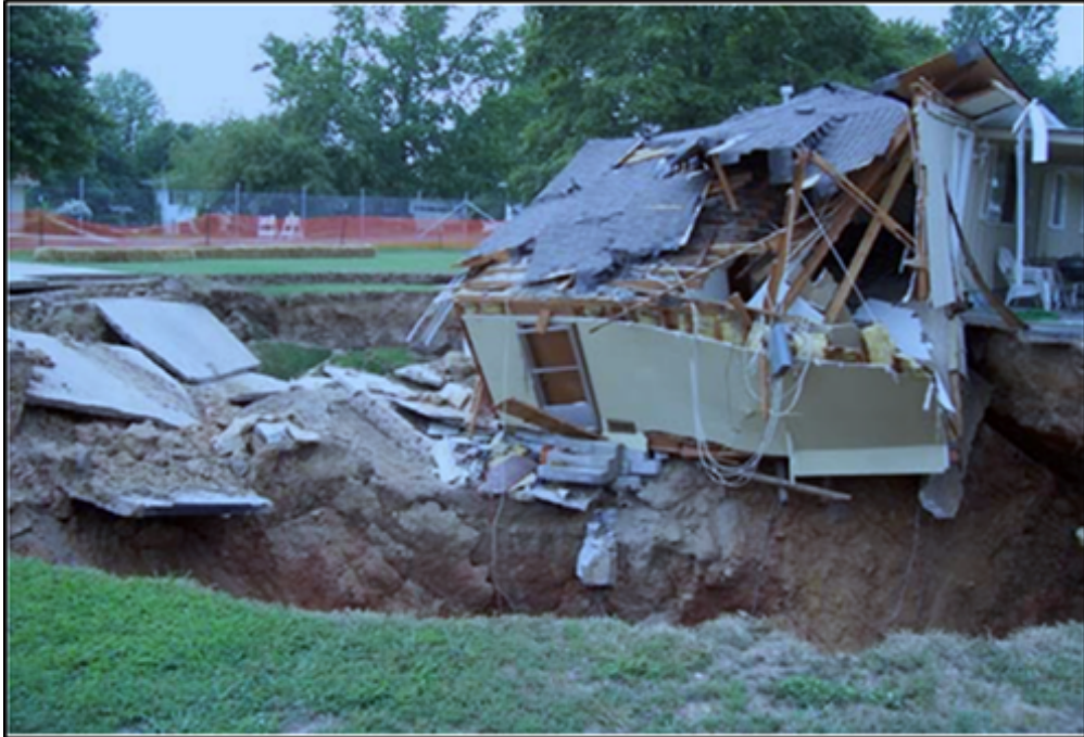
Figure 4.5. Sinkhole collapse that occurred in the southwestern Missouri town of Nixa which developed near the intersection of two nearly orthogonal solution-widened joint sets (Anderson, 2006).
