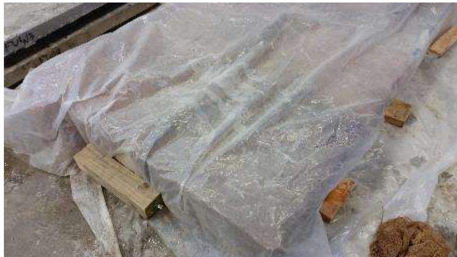
Figure 5.11. Plastic sheet on top of burlap
