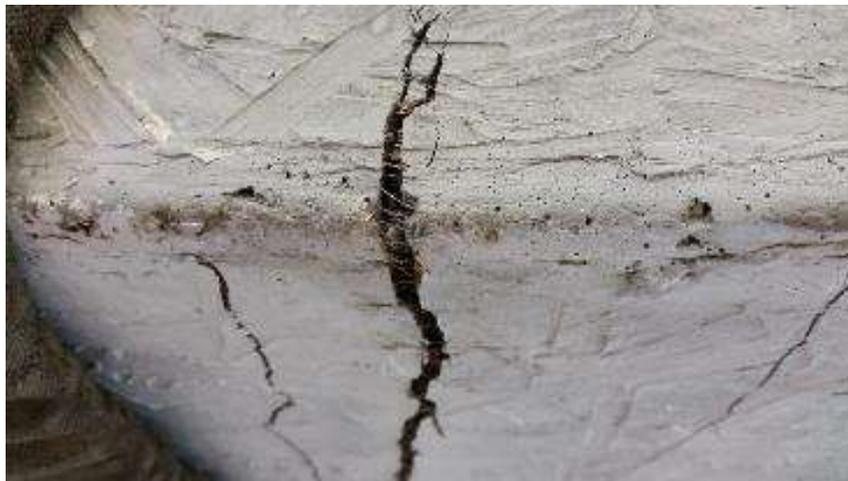
Figure 6.44. Tensile crack on panel SUN3
