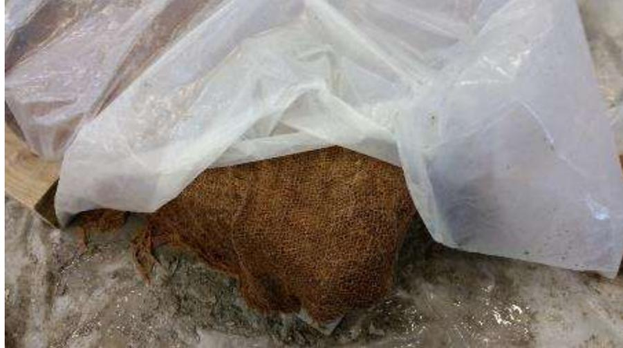
Figure 5.10. Wet burlap on top of concrete surface
