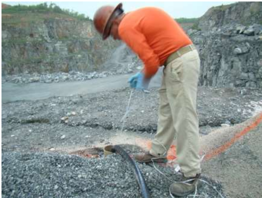
Figure 3.3. Loading a Hole for Test Blast 1 with Titan 1000 SME
