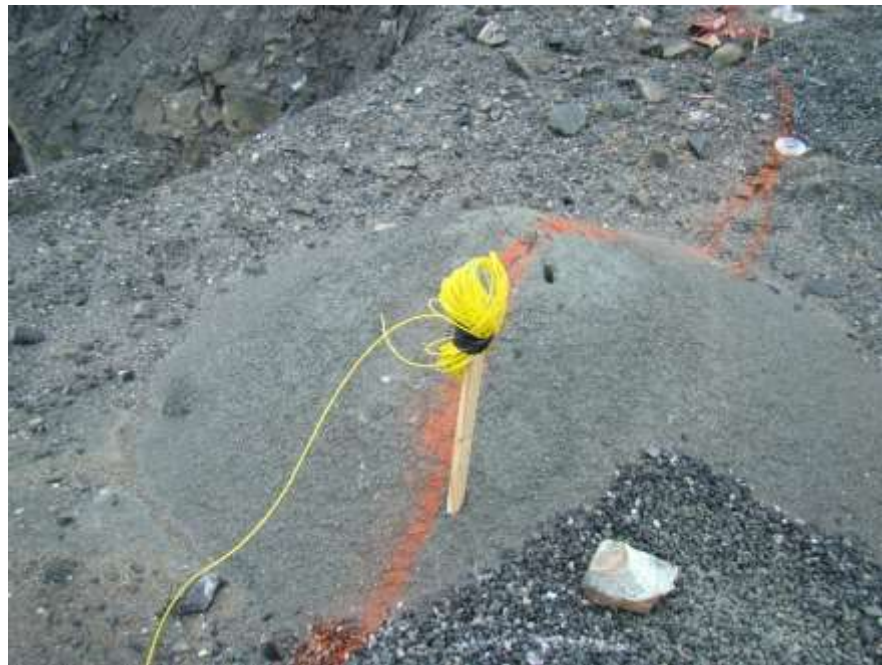
Figure 3.4. Shock Tube “Flash Bulb” (hole outside of photo in lower left)
