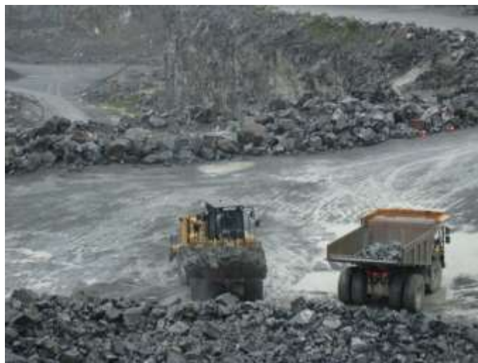
Figure 3.8. Shot Mucking (Catipillar 990 Loader)
