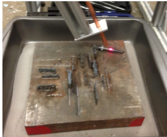
Figure 4.4. Laser welding process
