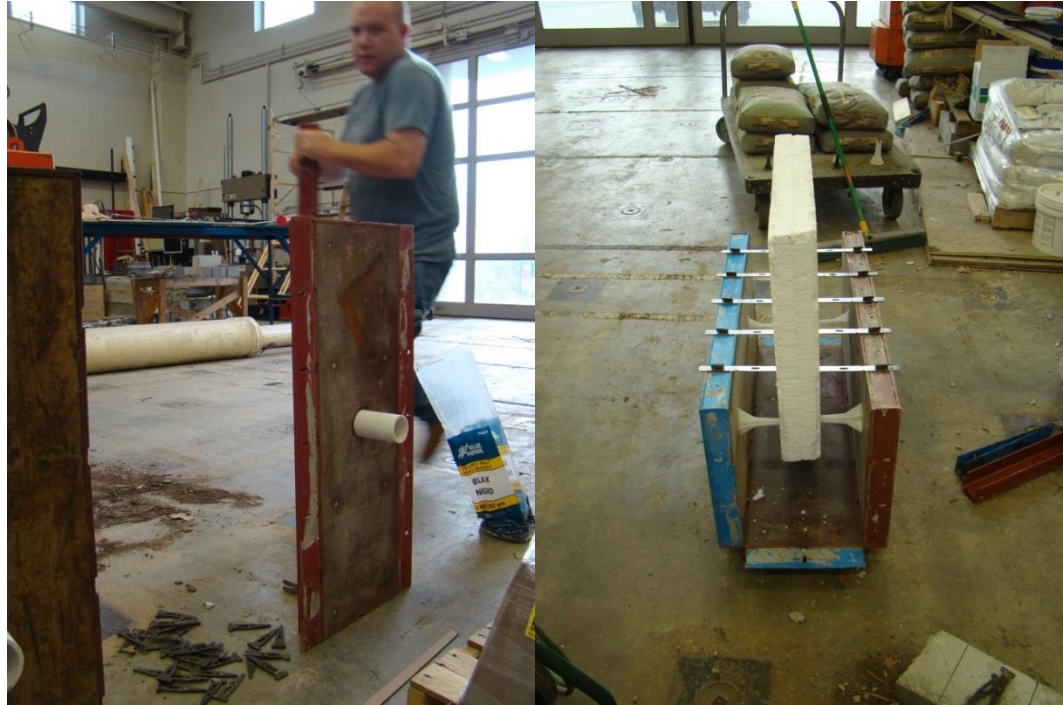
Figure 3.6 Construction of foam filler and framework
