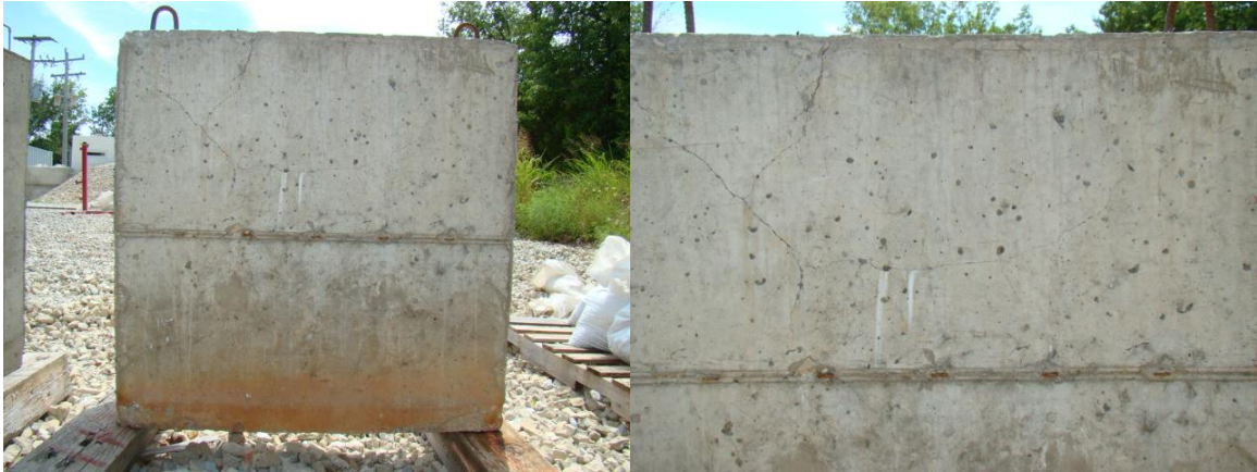
Solid concrete barrier
