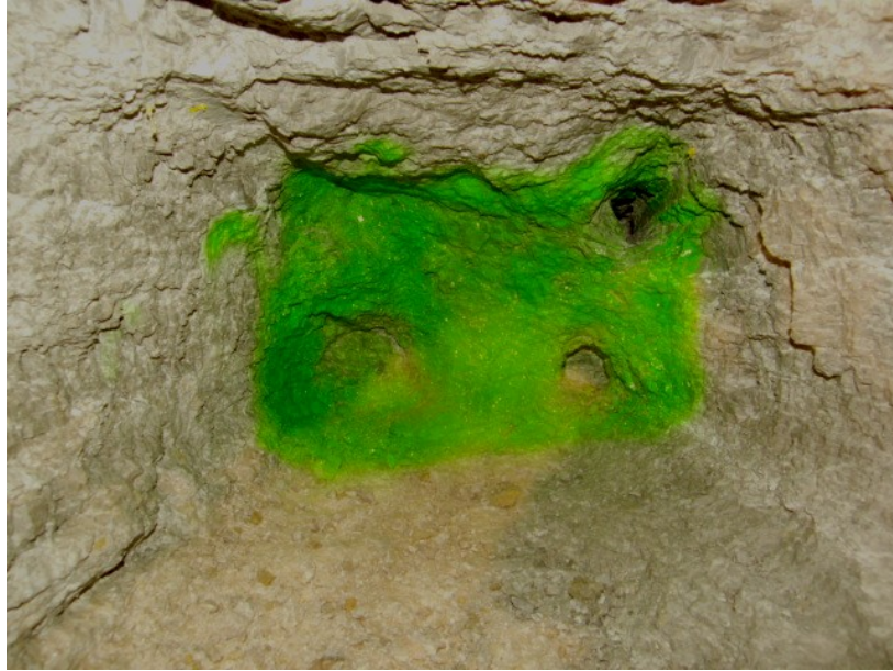
Figure 4.5. Typical Shortened Relief Hole Round (The resulting profile of Test 4 shows two bootlegs left by charged holes and one crater in the bottom left which represents the position of the last hole to fire. The back face of the cut has been painted green to accentuate its profile.)
