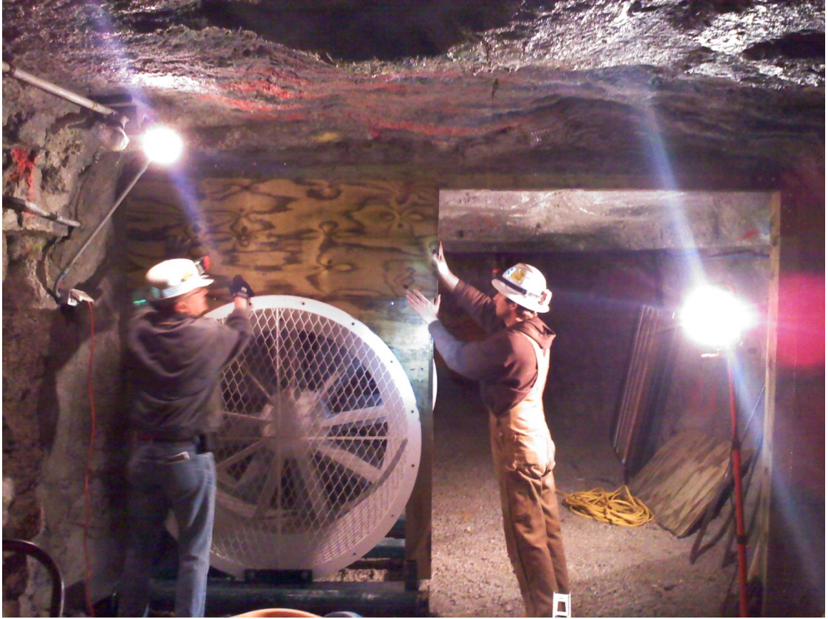
Figure 7.12. Blocking the area around the booster fan with 20mm plywood
