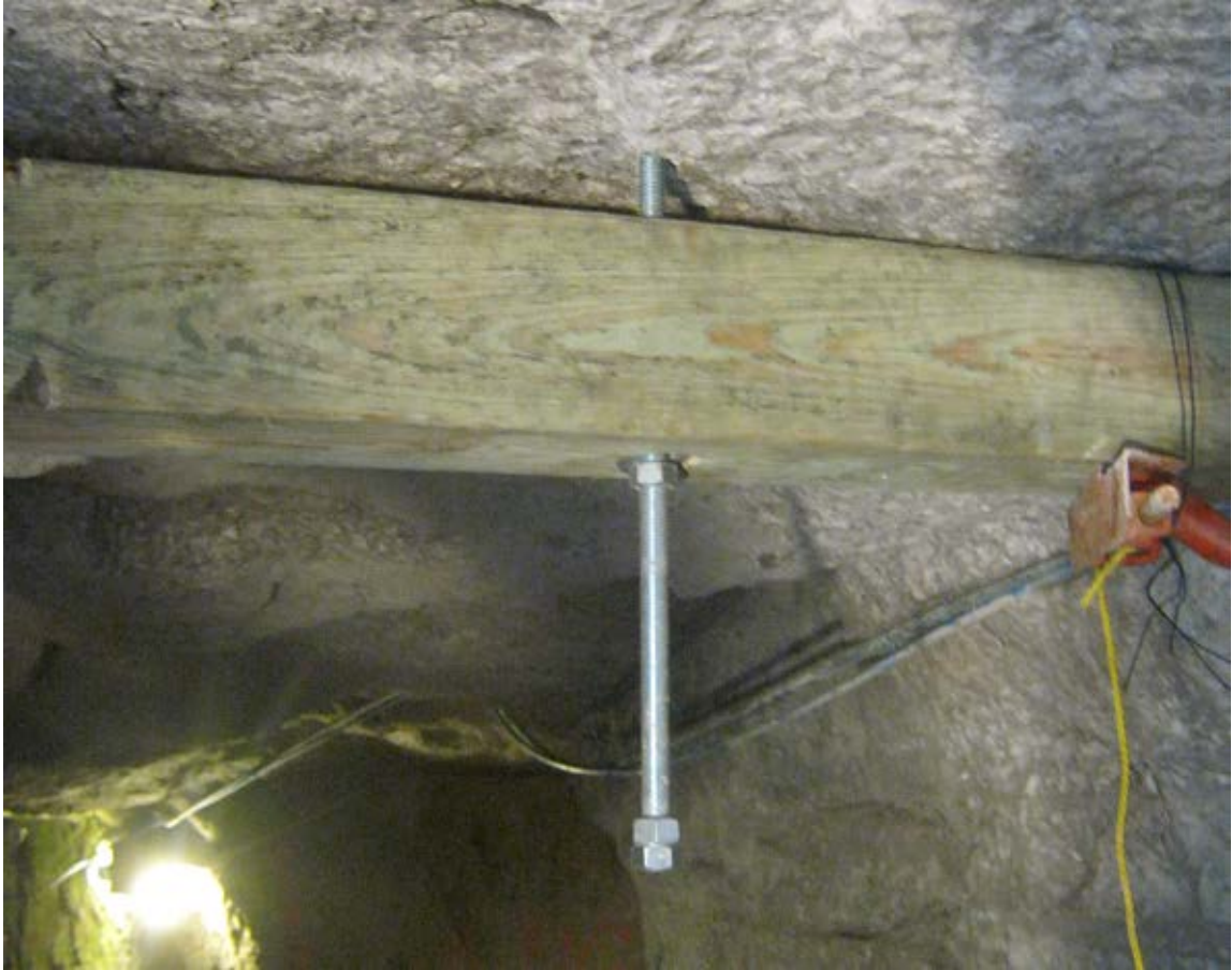
Figure 7.10. Anchoring the frame to the back of the mine
