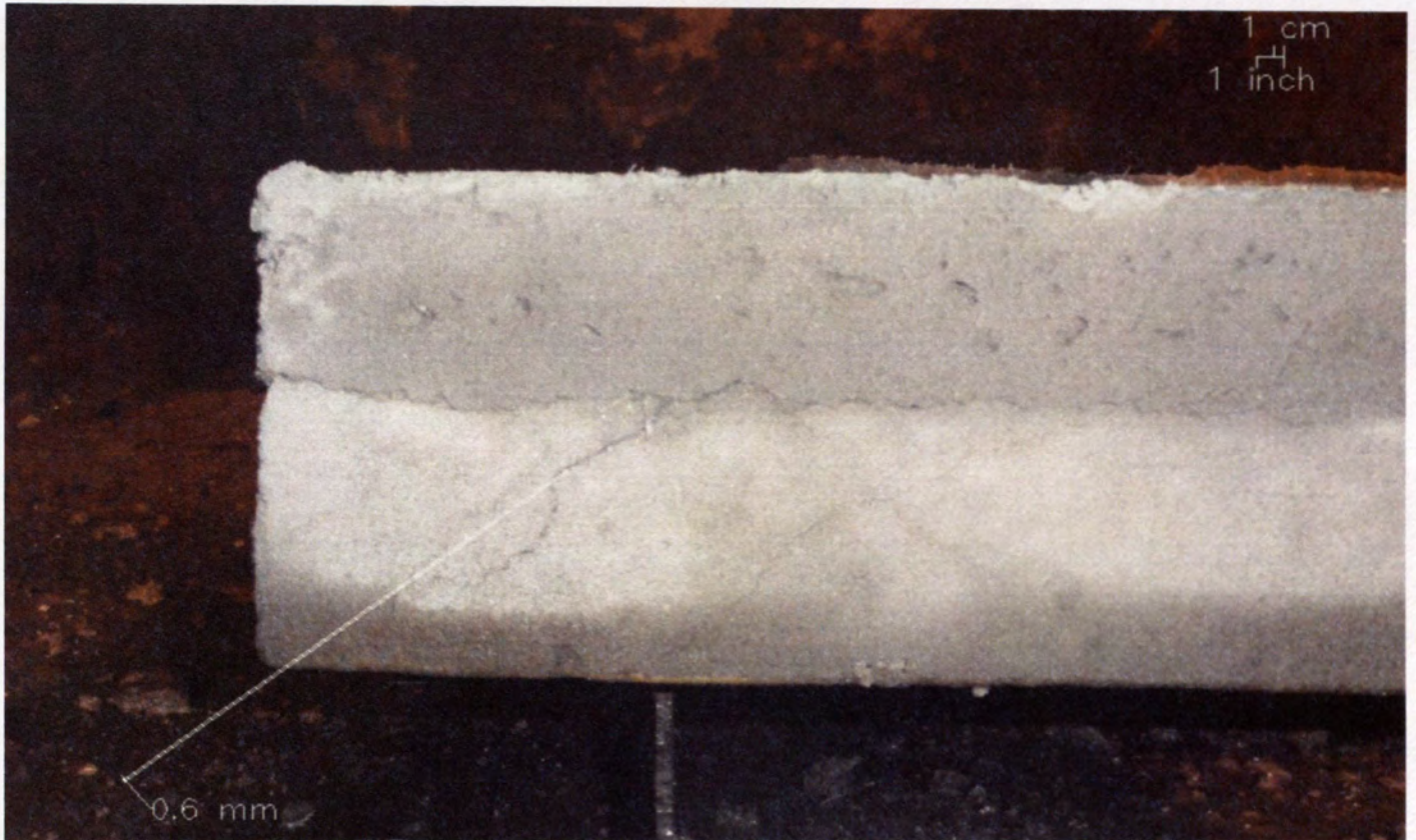
Figure E.14 – Shear Cracks in the Front Face of H-B, 1 st Event
