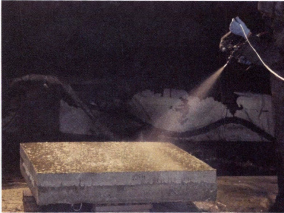
Figure 3.8 – E-Glass DFRP B Application
