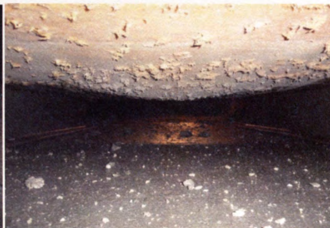
(f) Bulge in Tension Face
