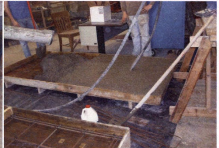
(b) Vibrating the Concrete
