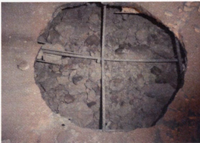
(e) Hole From Above the Panel
