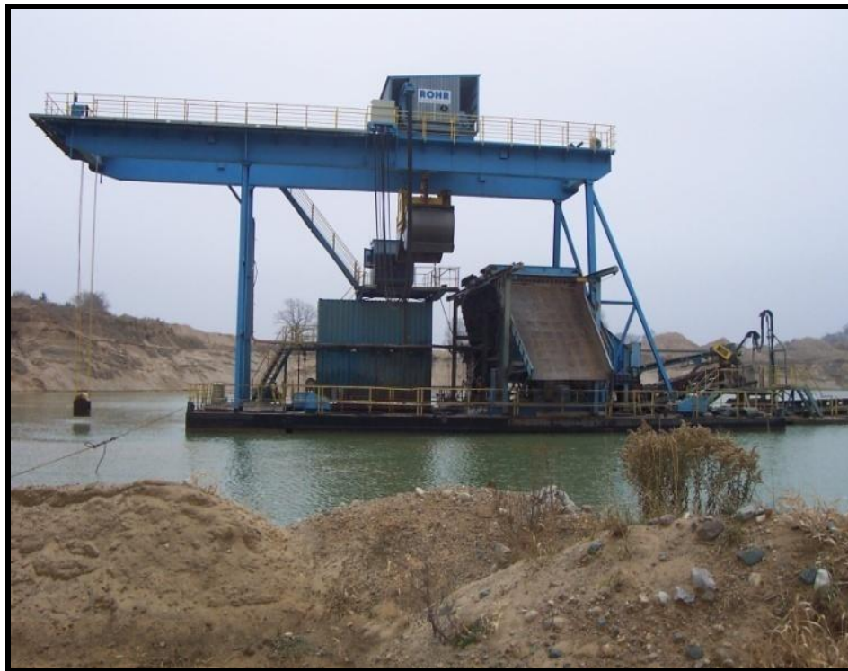
Figure 1.1 Clamshell dredge on site
