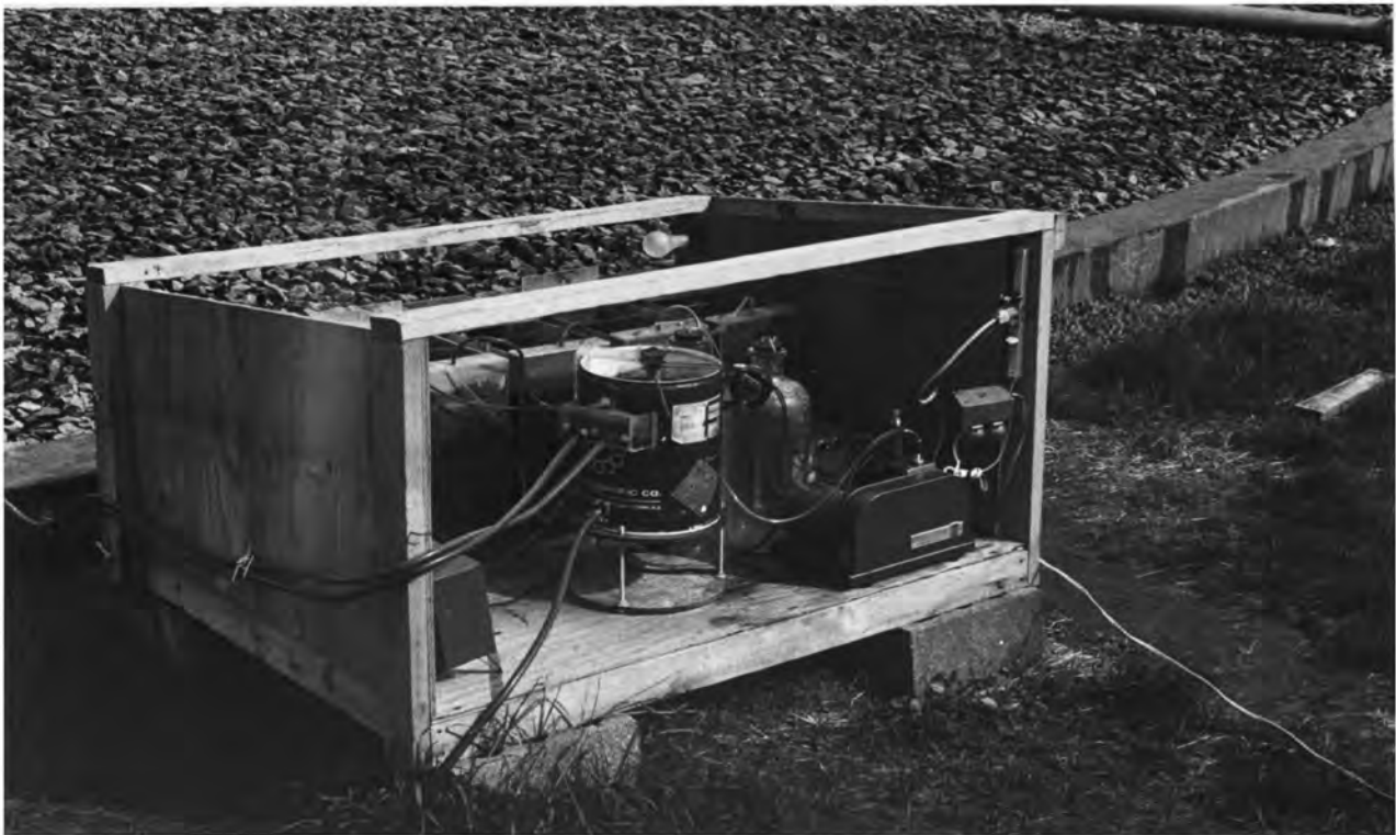
Figure 2. ACTIVATED SLUDGE PILOT PLANTS AND WASTE AND CHEMICAL FEED SYSTEMS
