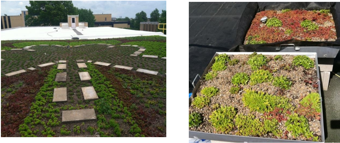
Figure 1.1. Built in place green roof on Missouri S&T's Emerson Electrical Engineering Hall (shown left) and modular roofing trays, Green Roof Blocks TM .
