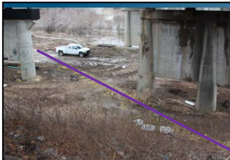
Figure 6.1. Data acquisition of profile 1
