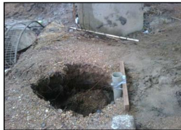
Figure 3.4. Karst feature near bridge pier at the project site
