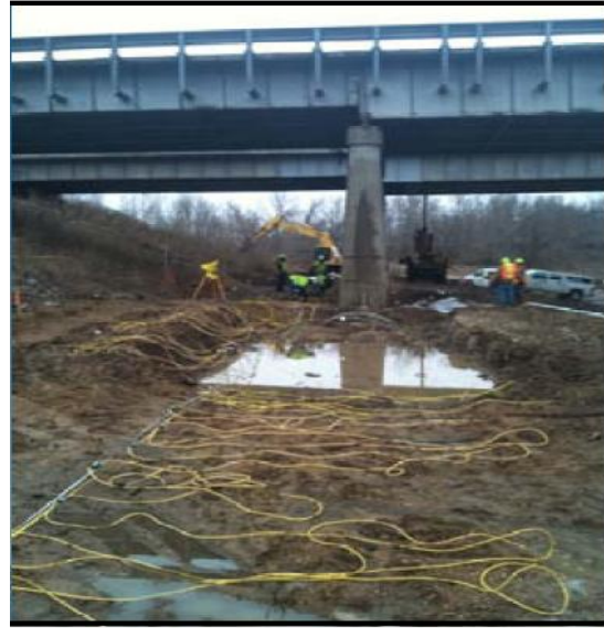
Figure 6.2. Data acquisition of profile 2
