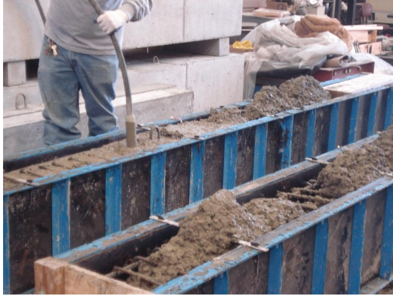
Figure 4.5. Internal Vibration
