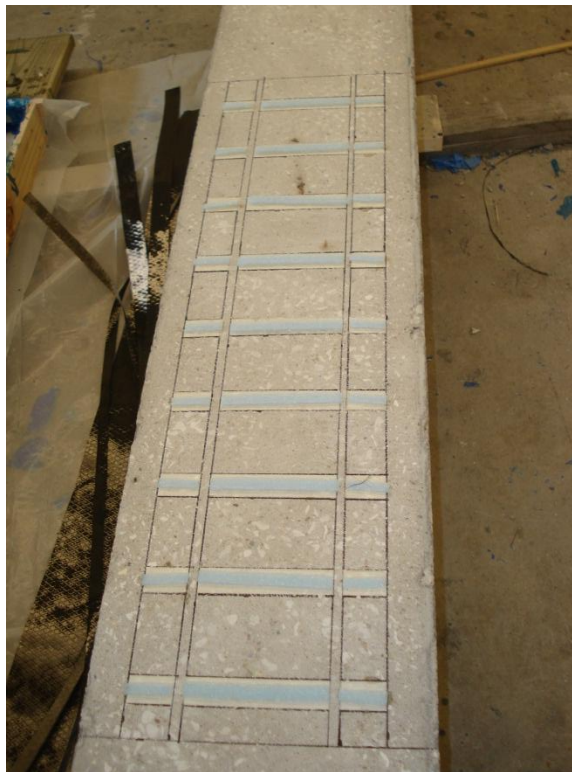
Figure 4.28. Layout of Foam Prior to FRP Application
