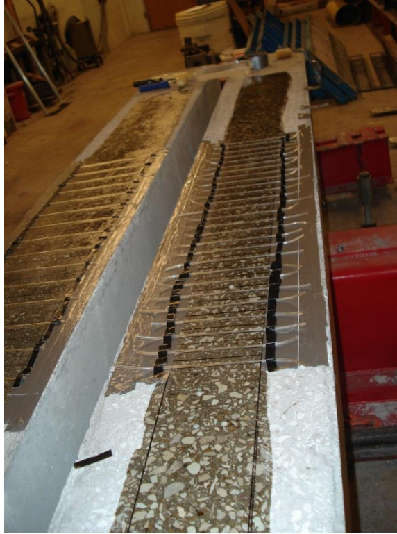
Figure 4.8. During FRP Application
