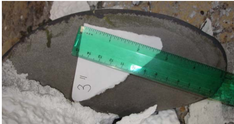
Figure 3.1. Oxidation on leading edge of propeller blade.
