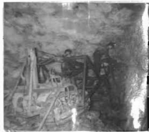
Fig. 4. Setting Up, Breast Hole.
