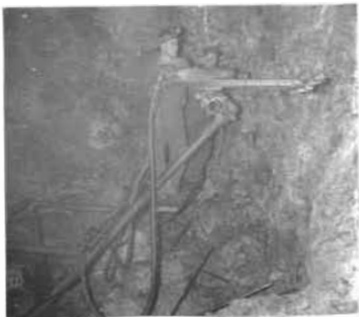
Fig. 2. Drilling a Roof Hole. With Automatic-Feed Short Sash Jumbo Machines
