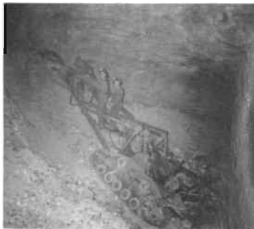
Fig. 3. Drilling in High Ground
