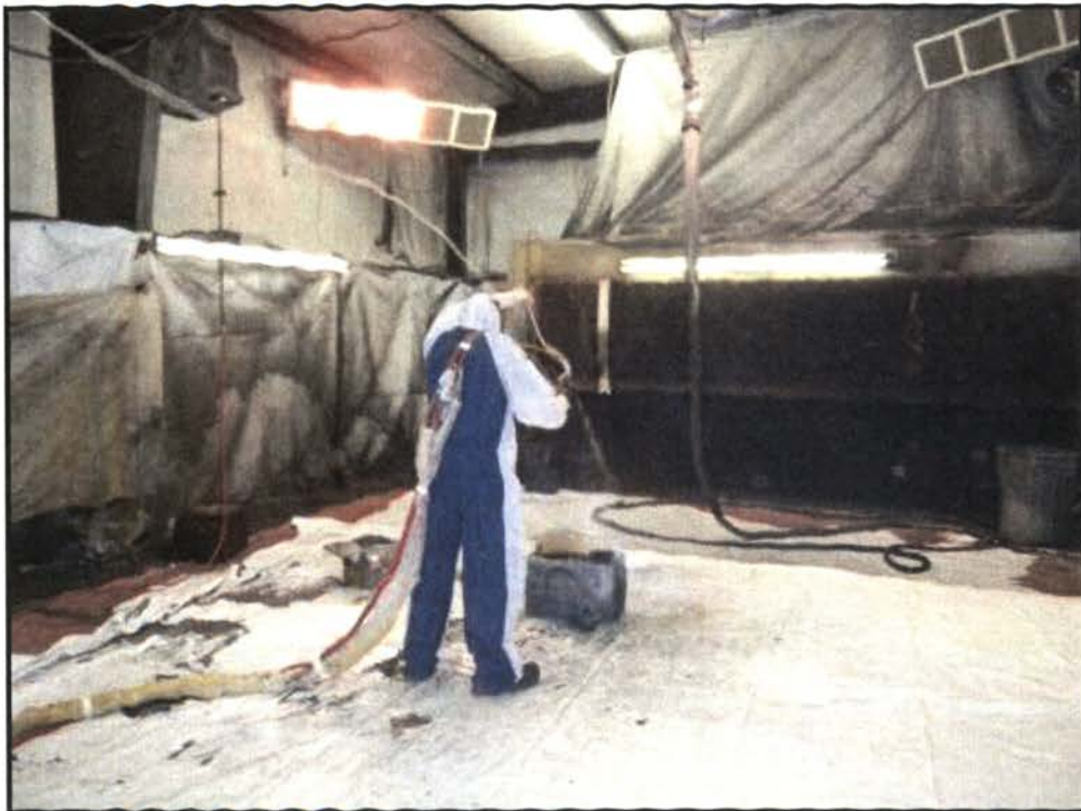
Figure 3.4. Polyurea-Fiber Spraying Process
