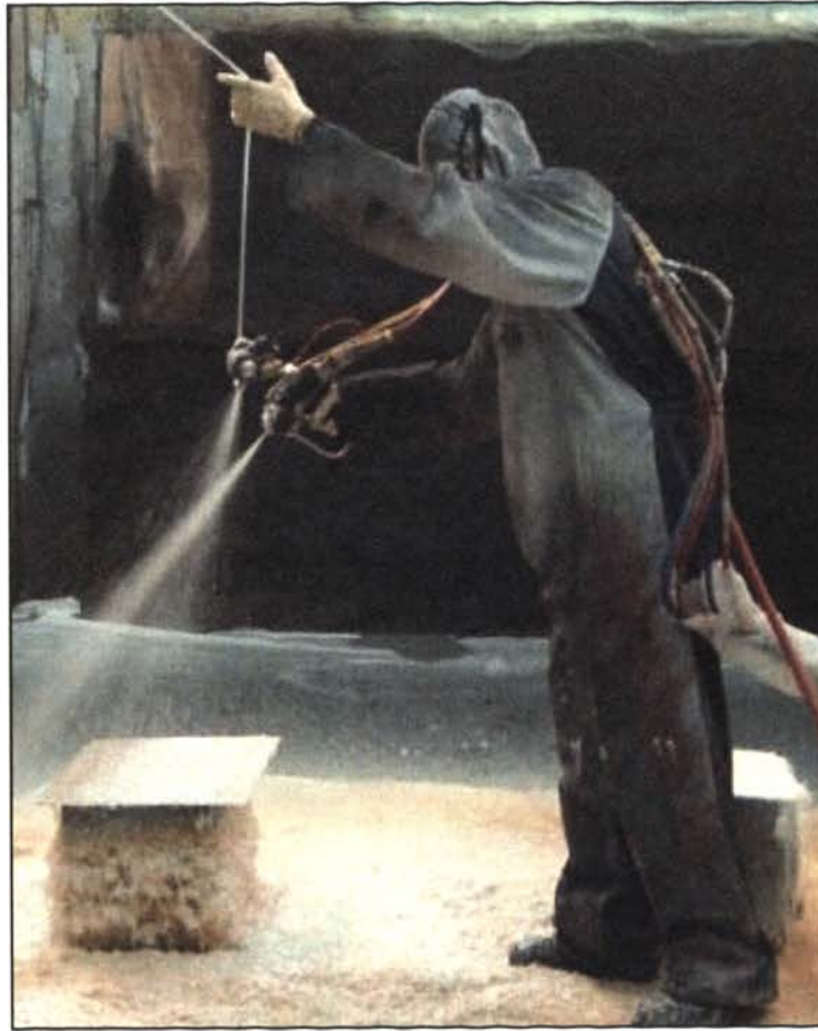
Figure 2.2. Polyurea-Fiber Application Process (Carey and Myers, 2010)
