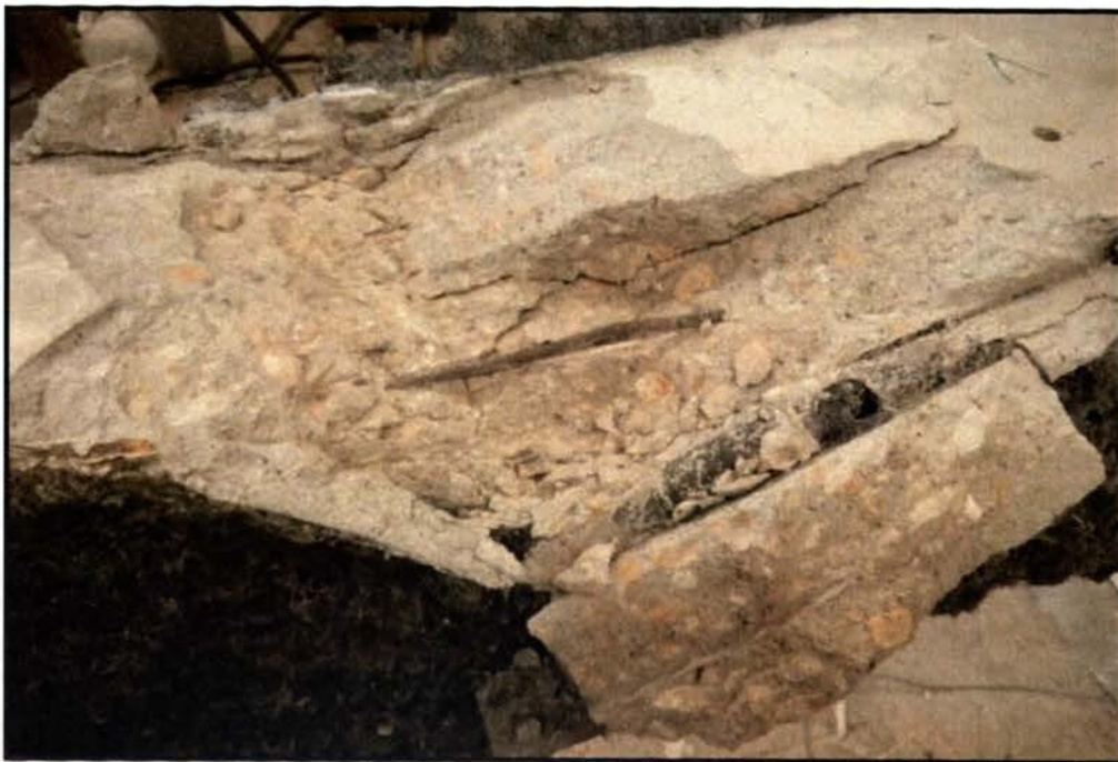
Figure 4.10. Side View of Failed Test Beam F-P-A-L
