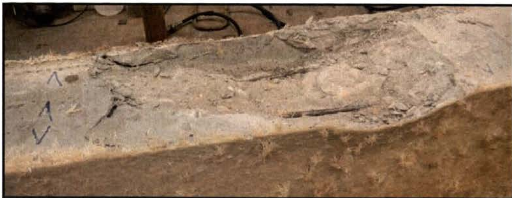
Figure 4.8. Side View of Failed Test Beam F-P-B-L
