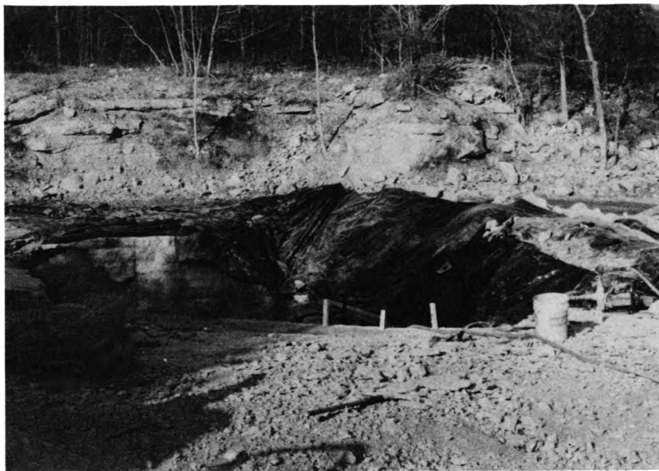
Figure 4. Typical Test Site Before Blasting.
