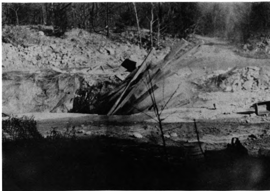
Figure 5. Typical Test Shot During Blasting.
