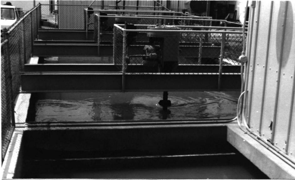
Figure 6. Neutralization Basin at Hoffman Taft Inc., Springfield, Mo.
