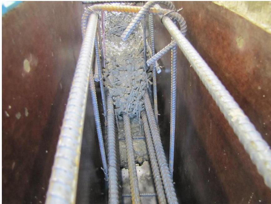
Figure 3.15. Concrete during placement into forms
