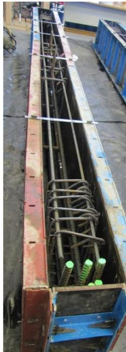
Figure 3.13. Reinforcing cage and formwork
