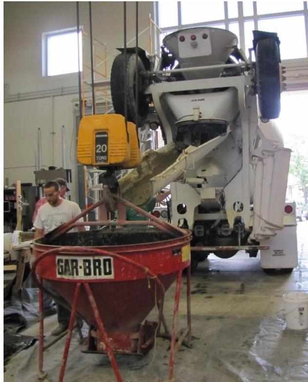
Figure 3.14. FRC transfer from concrete mixer to bucket
