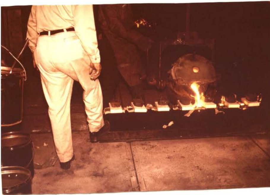
B. Pouring of molds from 100# ladle.
