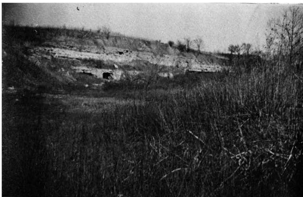
Quarry Face Winterset Limestone at top Bethany Falls Limestone at bottom Note:- Tunnel in Bethany Falls is 14 feet high.
