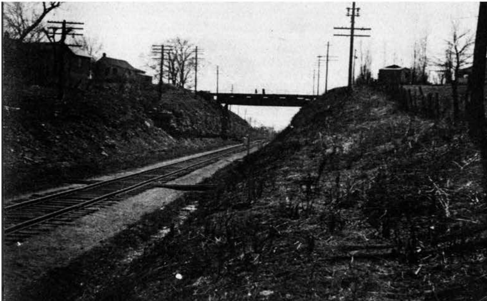
Cut in Iola Limestone SE part of Independence, Mo. on Missouri Pacific Railroad
