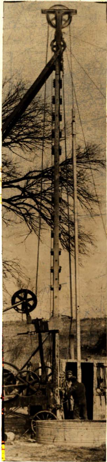
Drilling in the Blue Ridge Gas Field 107.
