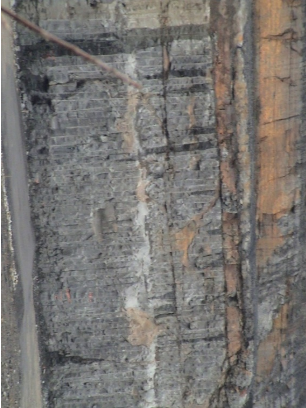
Figure 2.15 – Precision Presplit blast completed in 4 different rock types in Grundy, Virginia (Konya & Konya, 2017a)
