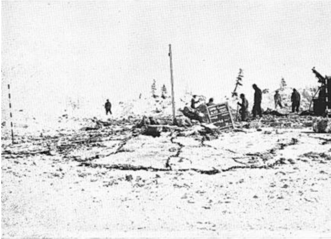
Figure 2.4 - Crater after Livingston (erroneously) showing shock breakage (Livingston C. , 1956)
