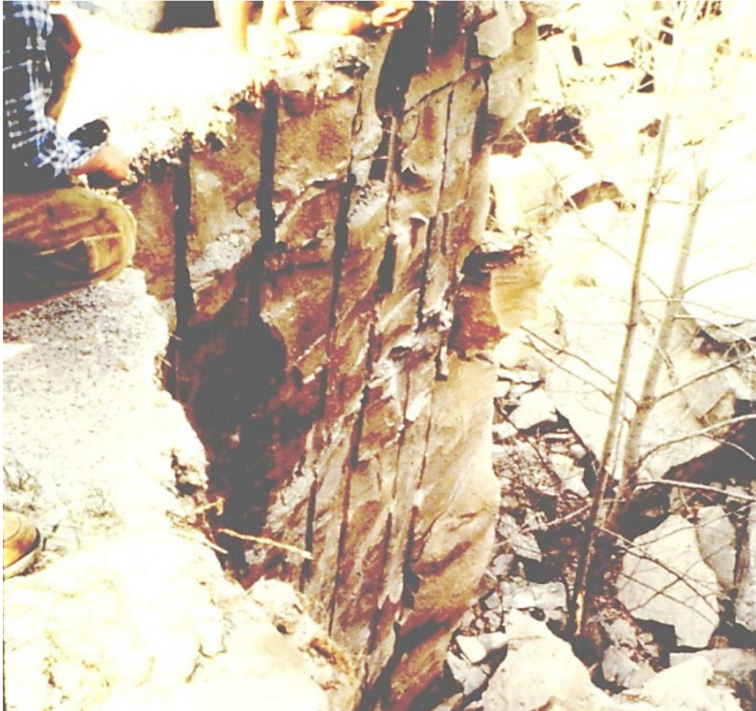
Figure 2.13 - First test of a Precision Presplit completed in 1980 (Konya & Konya, 2017a)
