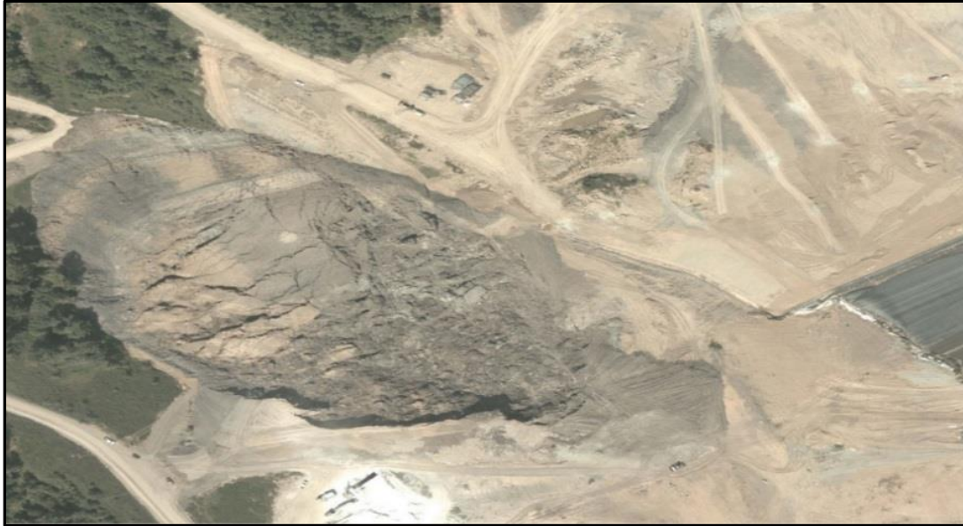
Figure 5.13: Aerial view of Big Run, KY landfill slide failure (source: https://kydep.wordpress.com/2014/04/24/what-does-an-8-acre-garbage-slide-look-like-big-run-landfill-slide-cleanup/ ).
