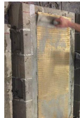
Apply fiber on matrix
