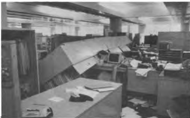
Fig. 28 Damage to Building Contents
