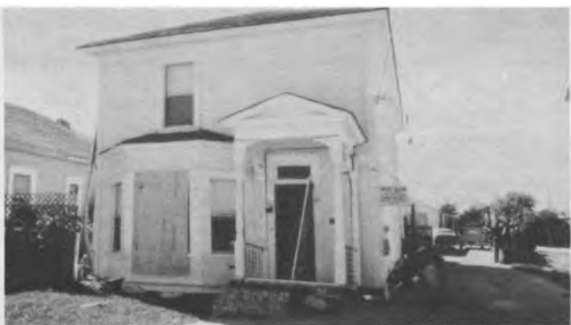
Fig. 4 Collapse of Home on "Pony" Walls
