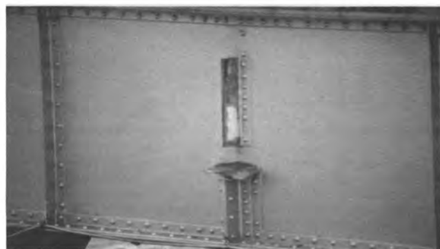
Fig. 19 Detail of Seat Connection on Bay Bridge
