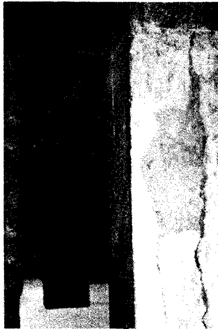
Photo 3 Surgical ward, Darbhanga (Cracks in r.c. column)
