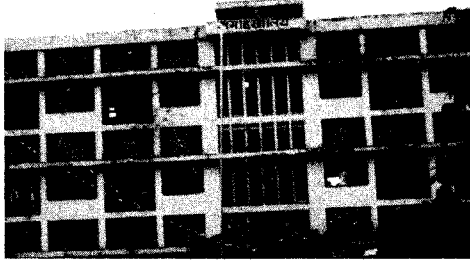
Photo 6 Collectorate Building, Samastipur (Walls showed heavy cracks)
