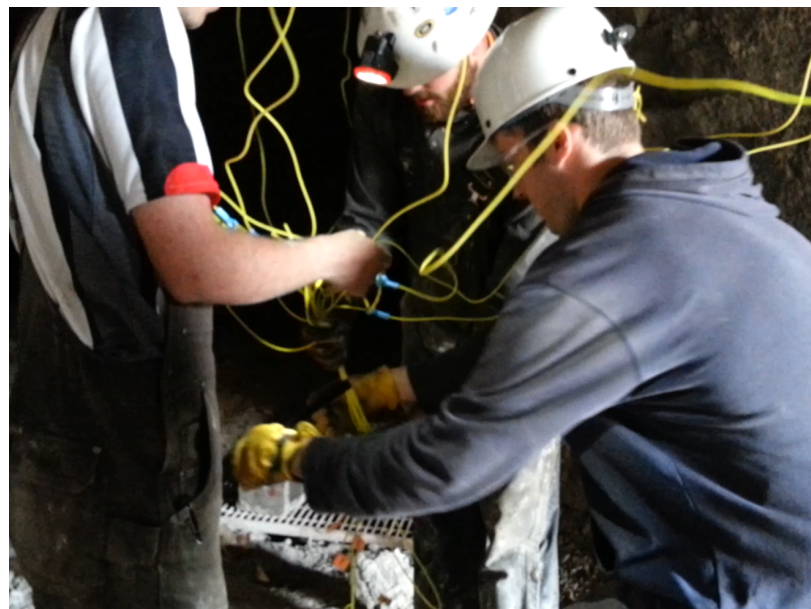
Figure A.4. Connecting individual detonating cords together
