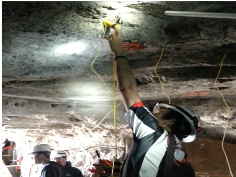
Figure A.3. Mounting the explosive material in to the mines surface
