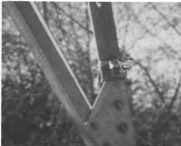
Fig. 9 Accelerometers glued at different locations on the pylon.
