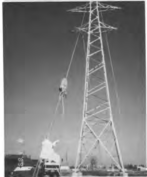
Fig. 16 Routine slacking test for the quality control of overhead line tower.
