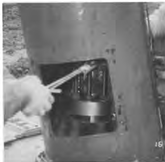
Fig. 7 Prestressing force tensioning.
