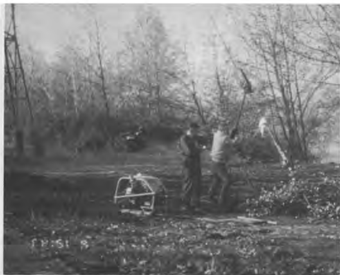
Fig. 10 Tensioning the cable for a slacking test.
