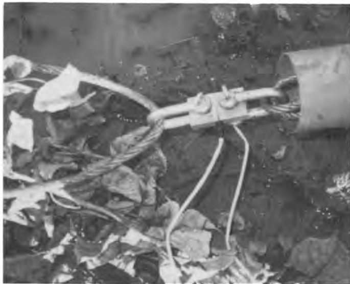
Fig. 11 Explosive tie allowing a sudden tension release.
