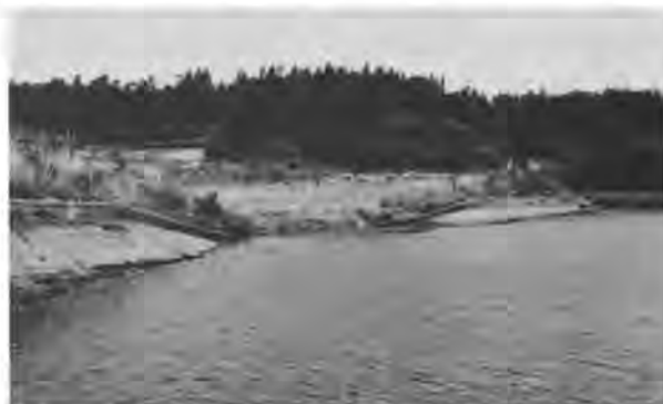
Fig.10 Kansuke Dam after Emergency Repair
