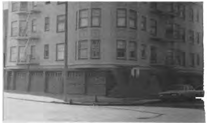
Figure 15. Marina district, San Francisco, October 24, 1989. View south west from junction of Scott and Alhambra showing damage due to shaking along Alhambra.
