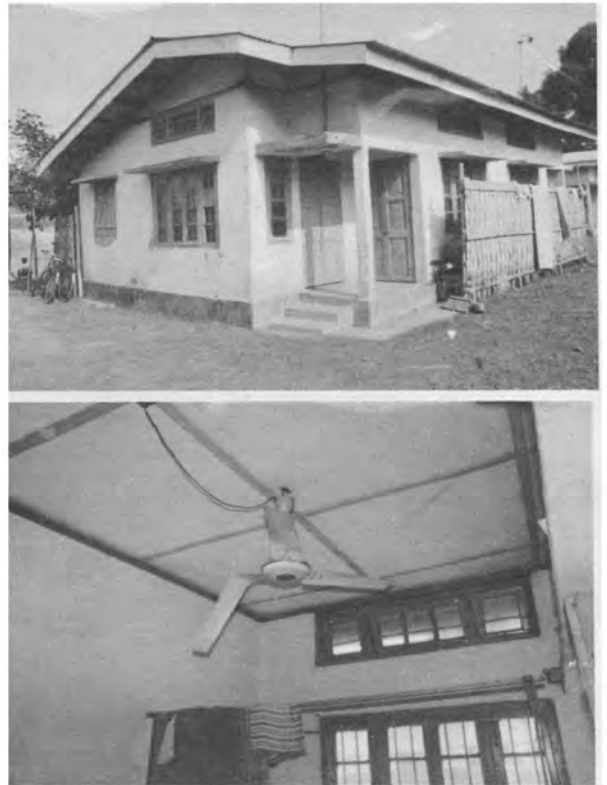
Fig. 2. Bending of blades of a ceiling fan in a building with reinforced concrete columns and beams, near the one in Fig. 1.
