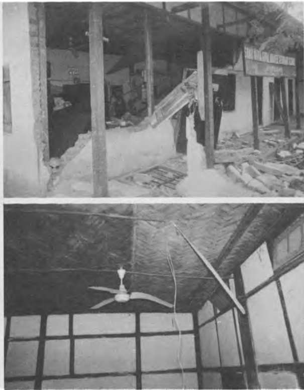
Fig. 1 Bending of blades of a ceiling fan in a timber frame building at Sonaimukh during Cachar earthquake.
