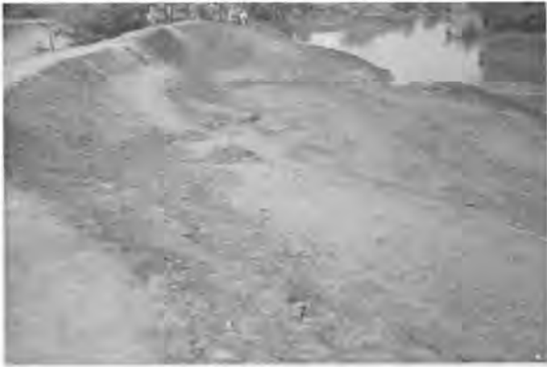
FIG. 7 Subsided Embankment of Kamala River.
