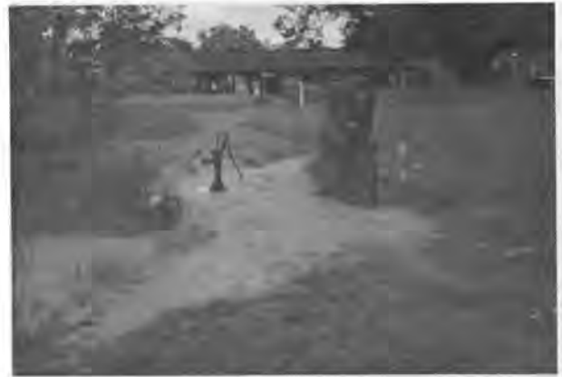
FIG. 3 Sand Boil, Around Hand Pump Inside the Residence of the Superintendent of Police, Darbhanga.
