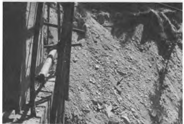
FIG. 13 The Landslide that Damaged the Tashiding Bridge (arrows show pieces of the suspension tower).
