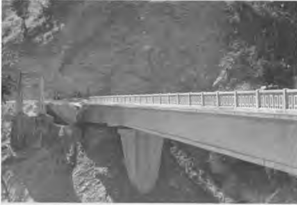
FIG. 10 A View of the Legship Bazar Bridge, Sikkim.
