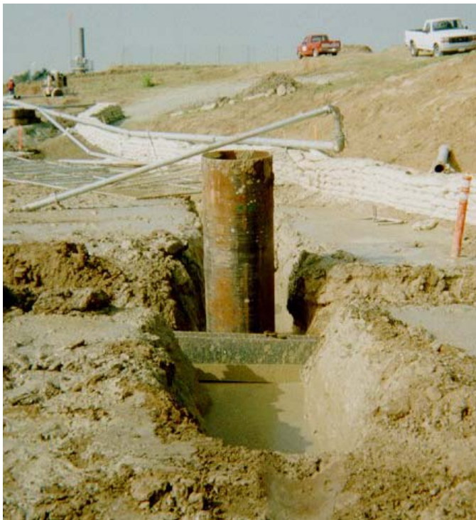
Fig. 7. Slurry wall construction between Upper and Lower Ramparts.
