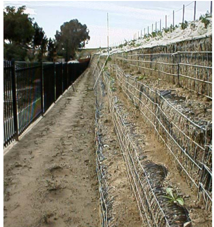
Fig. 12. MSE wall on the south side of Lower Ramparts immediately following the end of construction.
