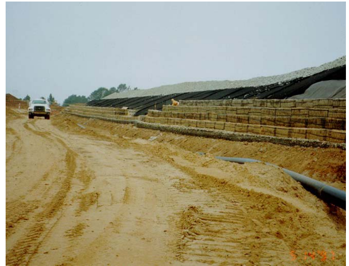
Fig. 13. The MSE wall between Lower and Upper Ramparts under construction.
