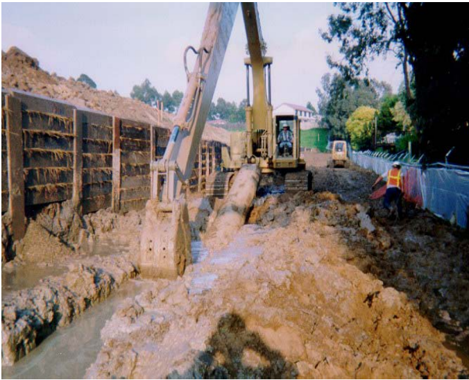
Fig. 11. Slurry wall construction along the south side of Lower Ramparts.
