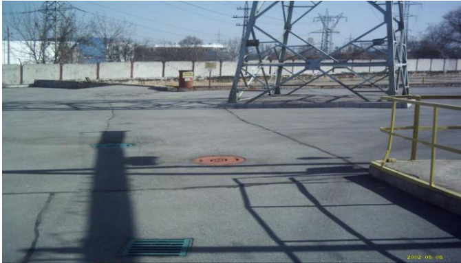
Photo 1: Rolling and steel poles for high voltage
