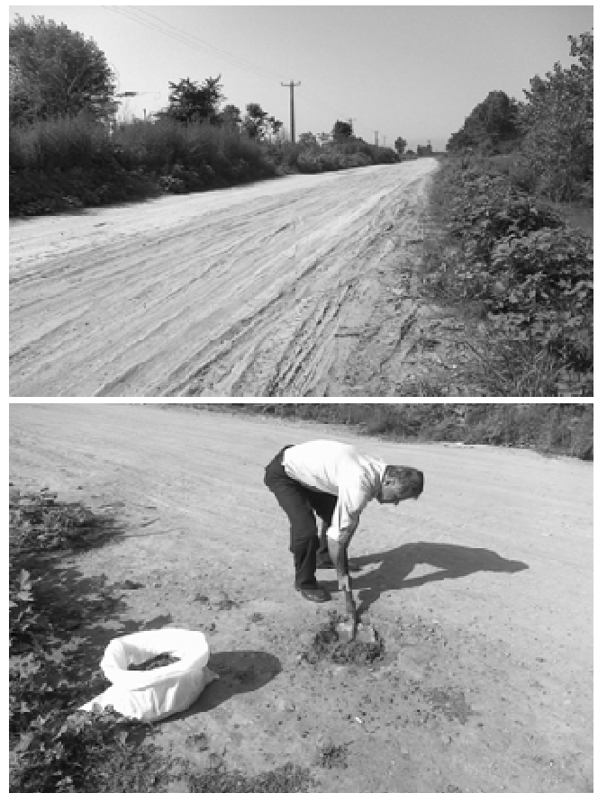
Fig. 1. Extracting the weak soil from Boodian road in North of Iran
