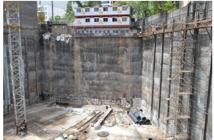
Fig. 7. Excavated and Stabilized walls of Rosha Trade Complex
