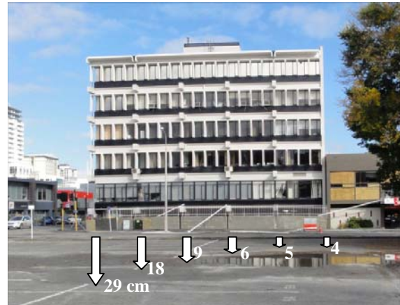
Fig. 12 Liquefaction-induced differential settlement of a CBD building on shallow foundations
