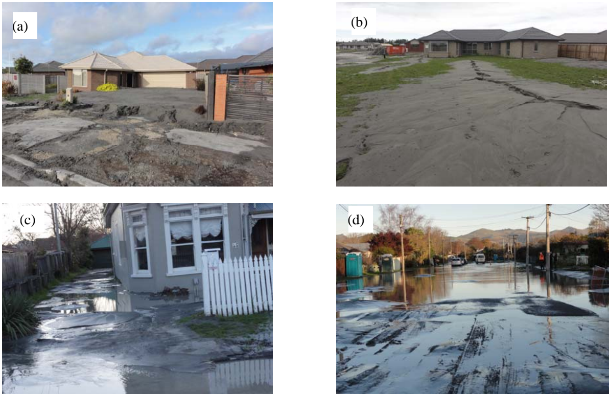
Fig. 5 Severe liquefaction in residential areas (suburbs along Avon River in the abandoned “red zone”)
