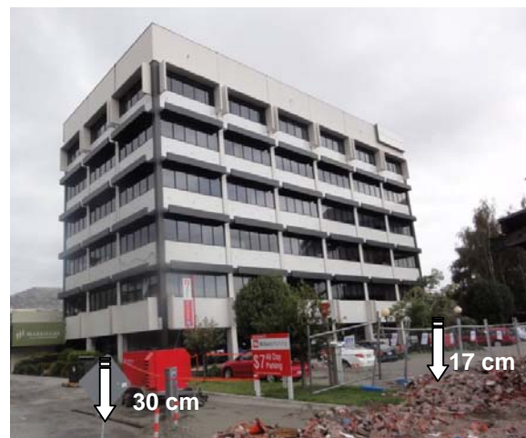
Fig. 12 Liquefaction-induced differential settlement of a CBD building on shallow foundations
